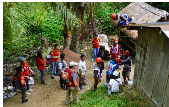
Figure 1 Strengthening of houses
